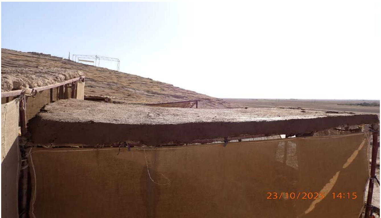
Figure 28: Applying thin mud plaster on the protective system of one wall without removing the old plaster
