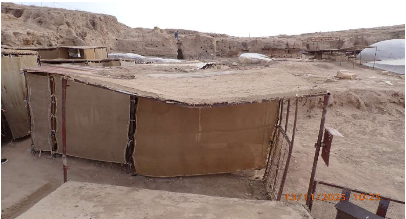
Figure 20: Bent metal rod at the opening of the south wall of Room C3
