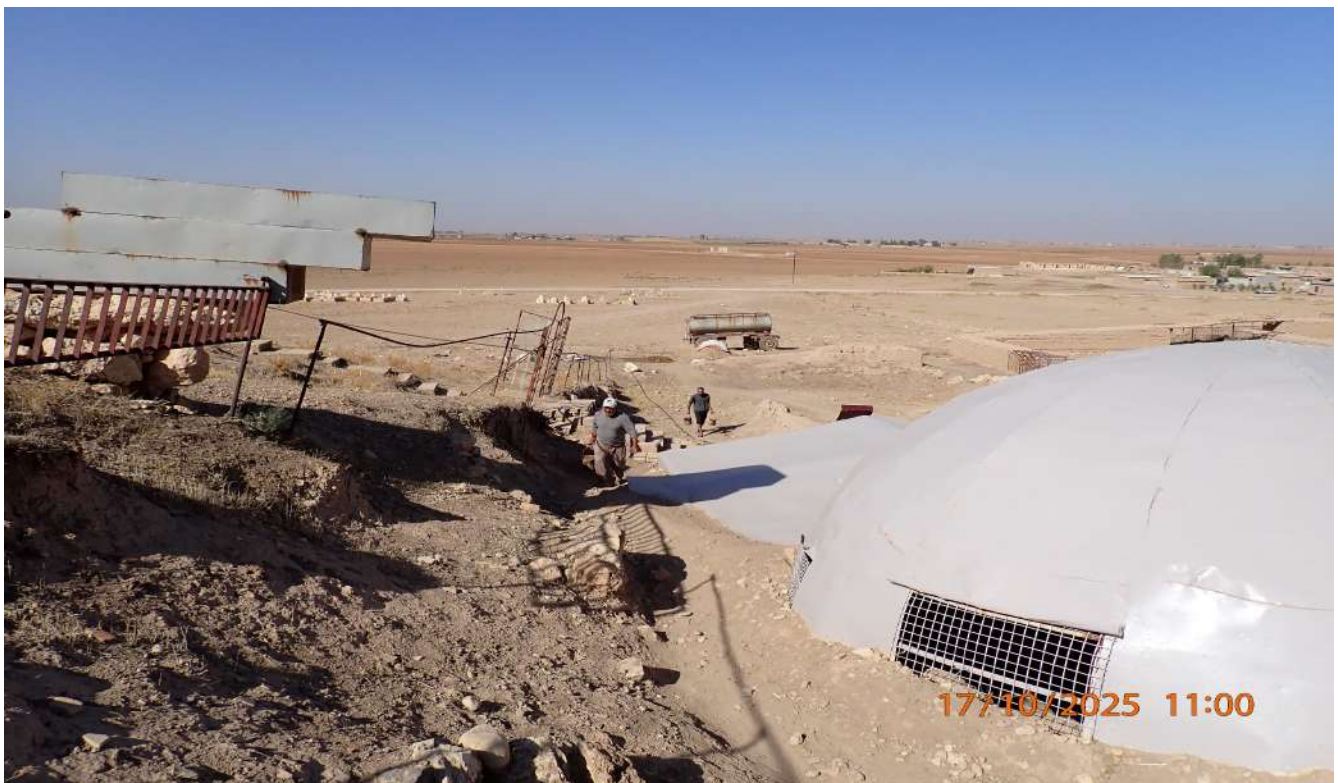
Figure 10: Long distance between work area and the mud plaster preparation area
