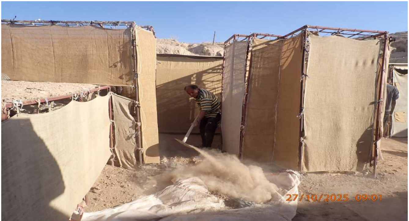
Figure 13: Collection of the debris
