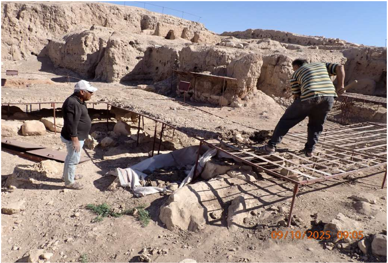
Figure 11: Removal of the fragile and deteriorated mud plaster
