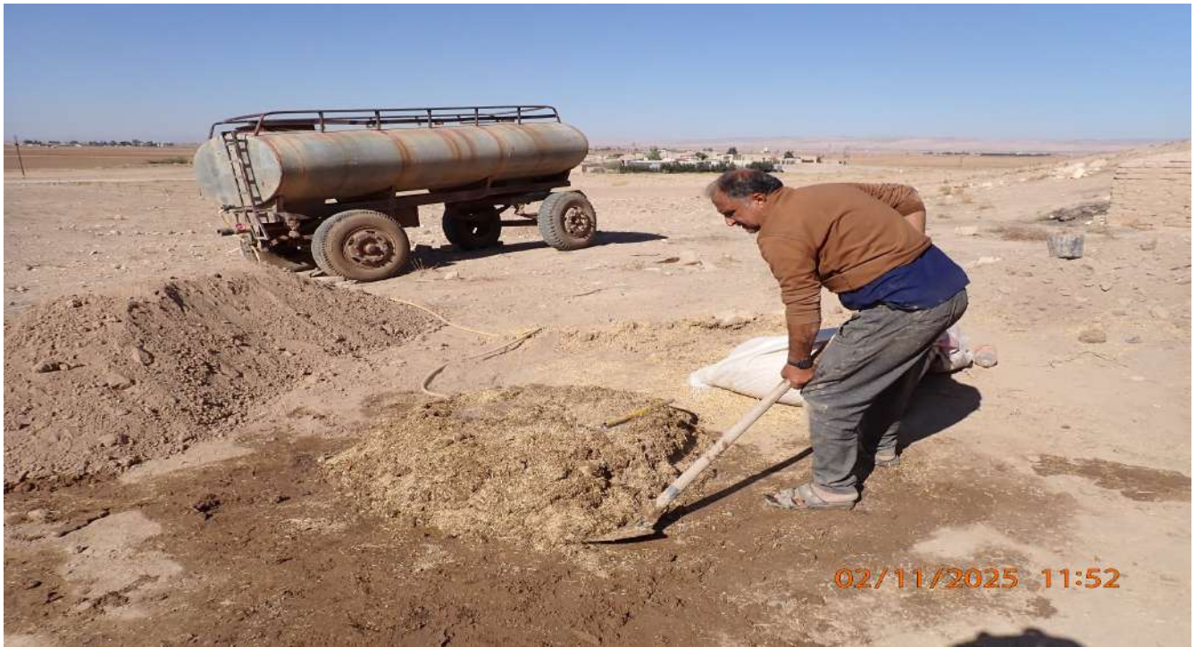
Figure 23: Mud plaster preparation
