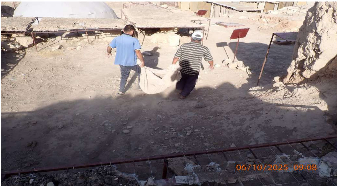
Figure 14: Debris transported away from the excavation areas
