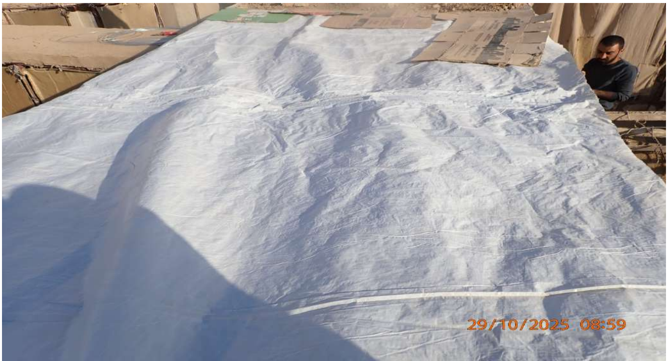
Figure 16: Placement of plastic sheet
