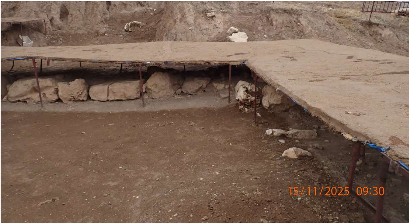
Figure 4: Some walls surviving only at the foundation level
