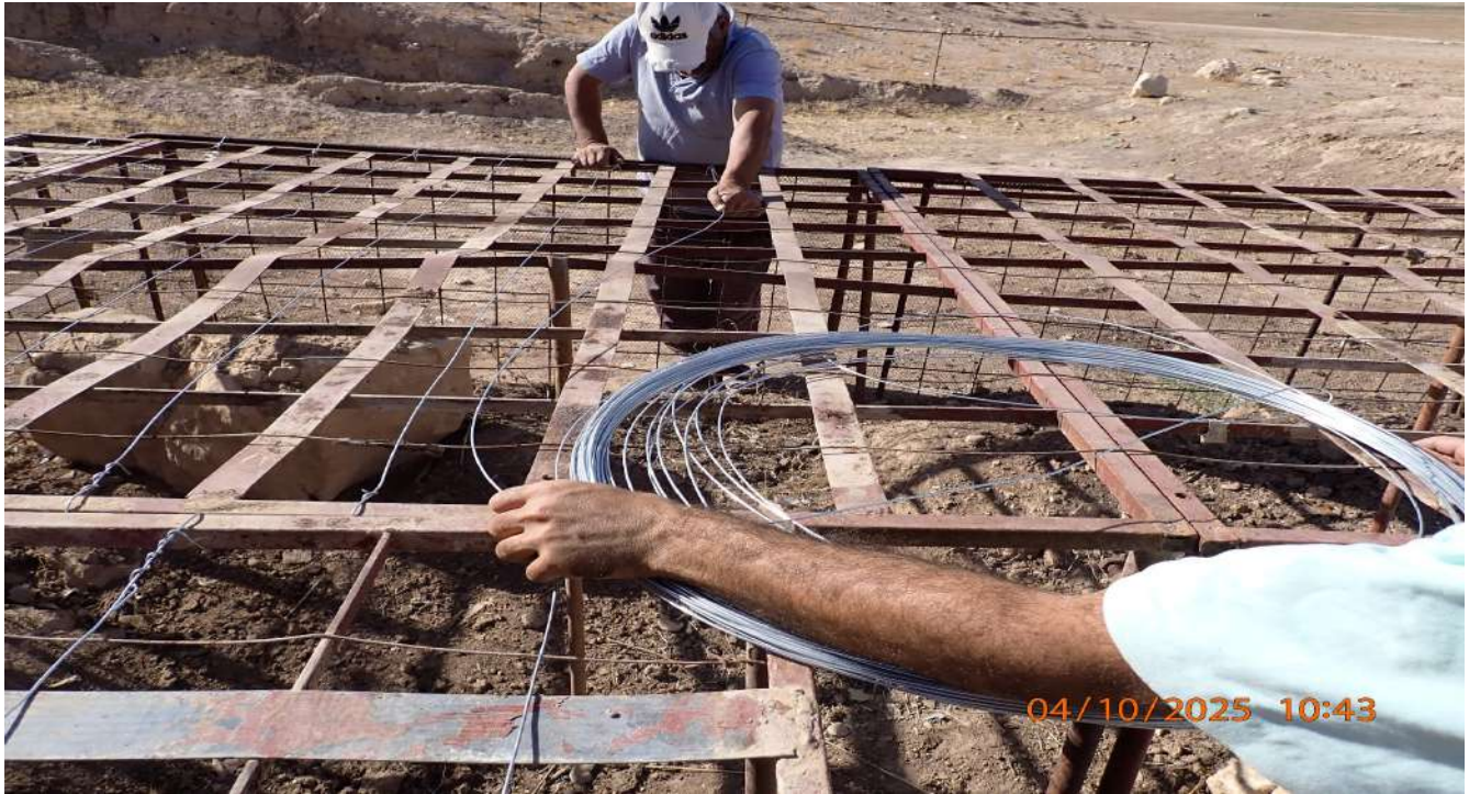
Figure 15: Metal wires installation
