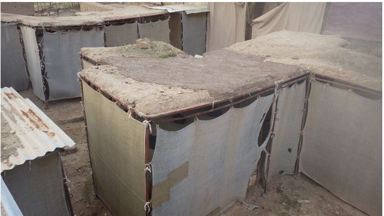
Figure 6: Reapplying thin surface plaster layers to the protective system surfaces
