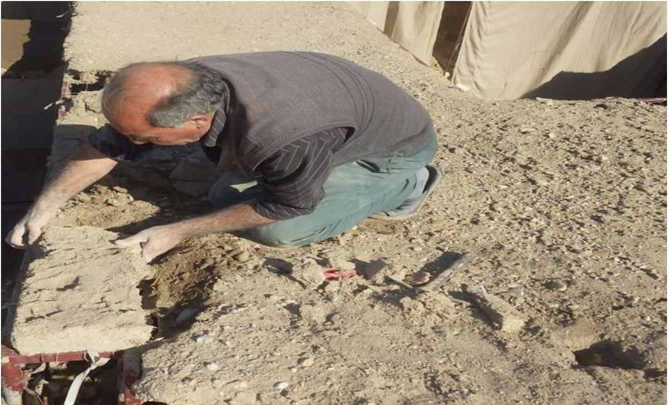
Figure 5: Sealing the gaps on the surfaces of the protective systems
