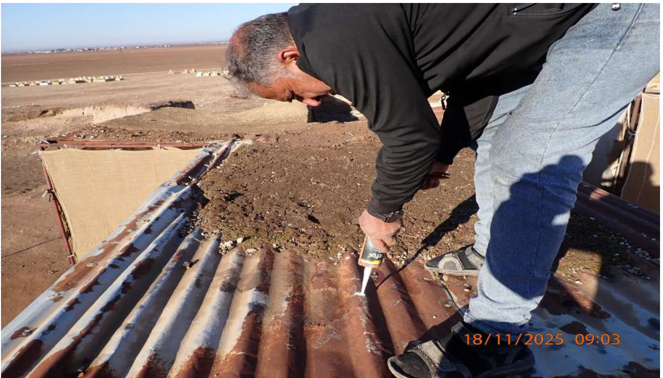
Figure 30: Sealing gaps and existing holes in sheet metal (tutiya) with silicone
