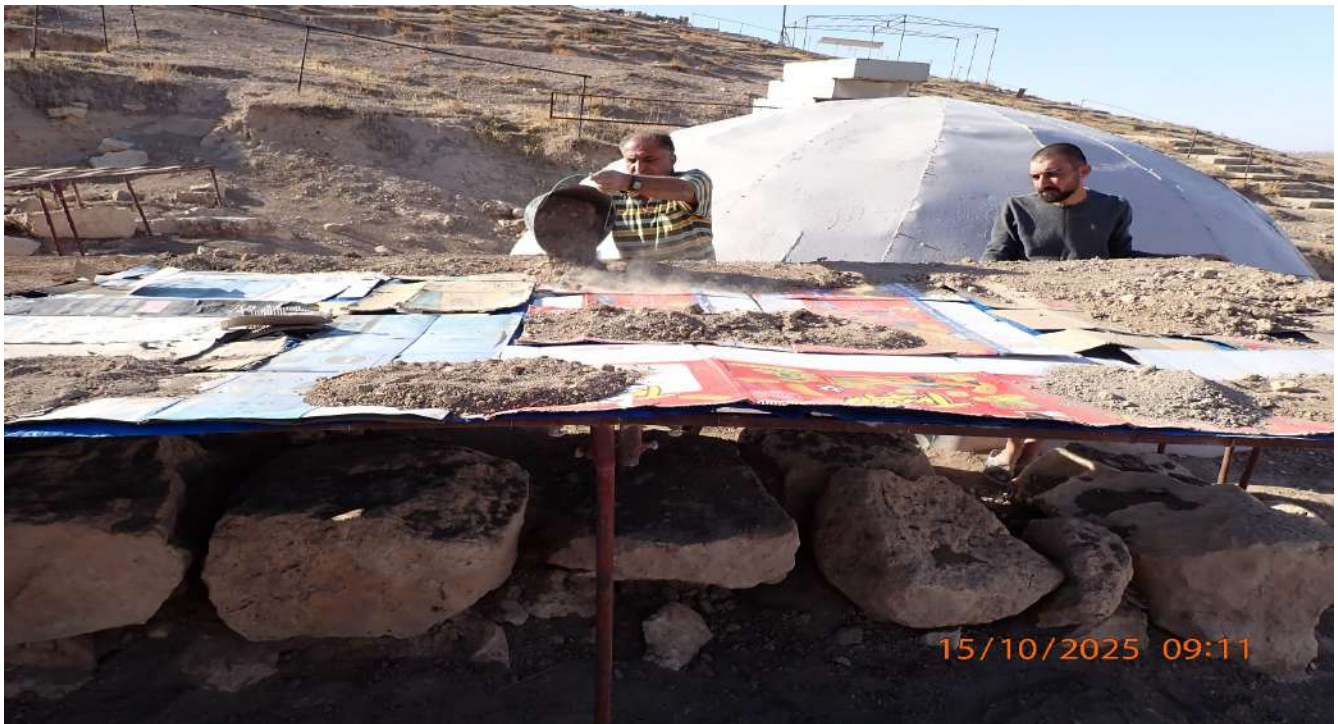
Figure 19: Applying a layer of soil from the old mud plaster
