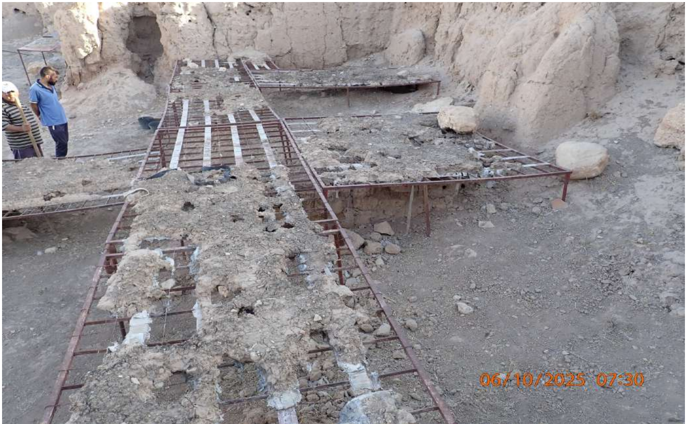
Figure 9: Patchy and inconsistent mud plaster on protective shelters in sector H
