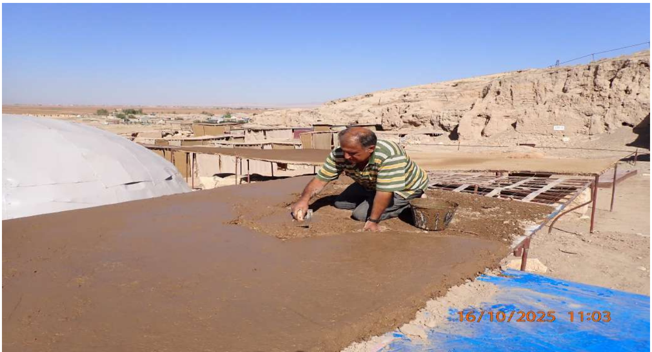
Figure 24: Application of a thick plaster layer
