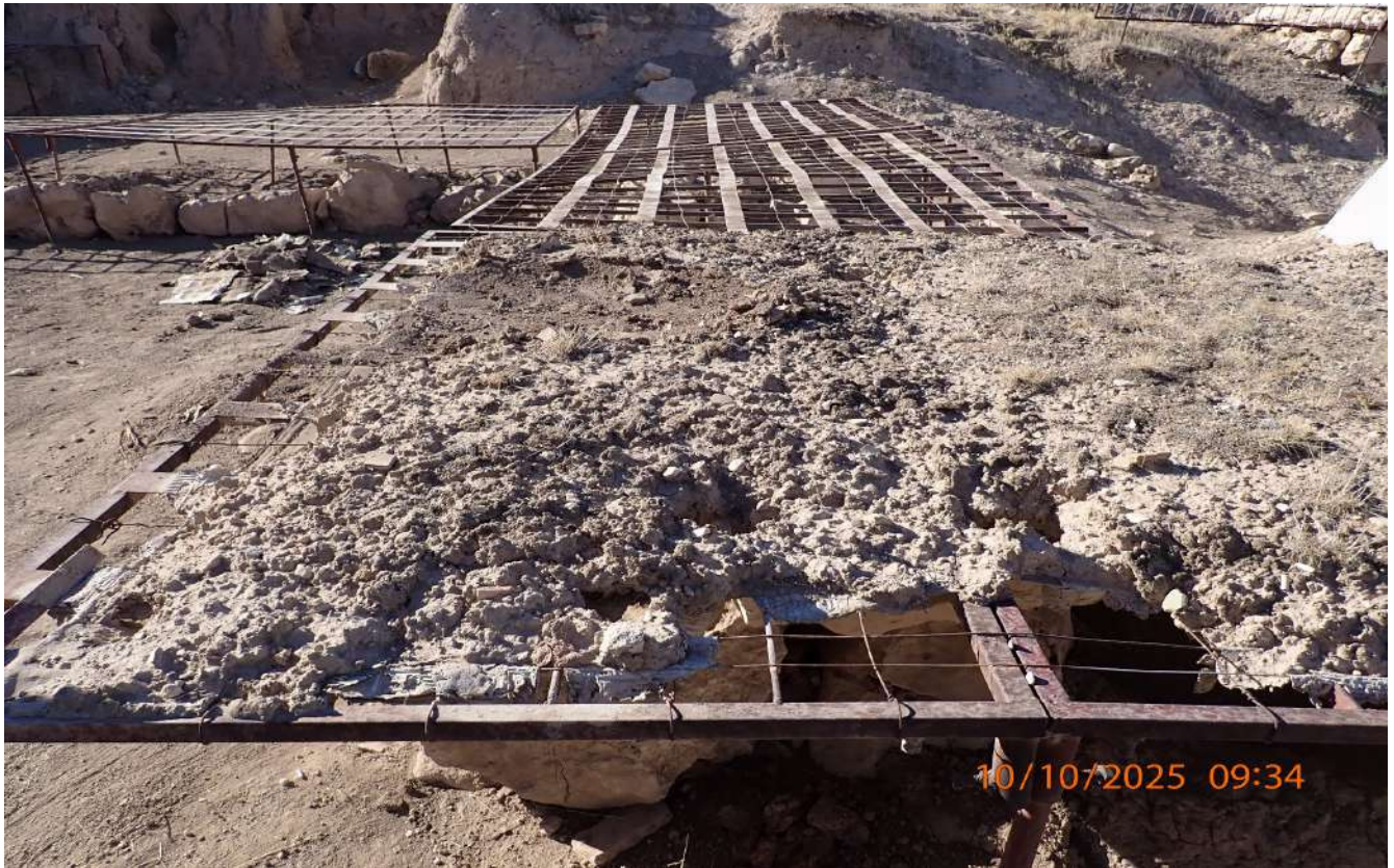
Figure 7: An image showing the fragile and detached mud plaster
