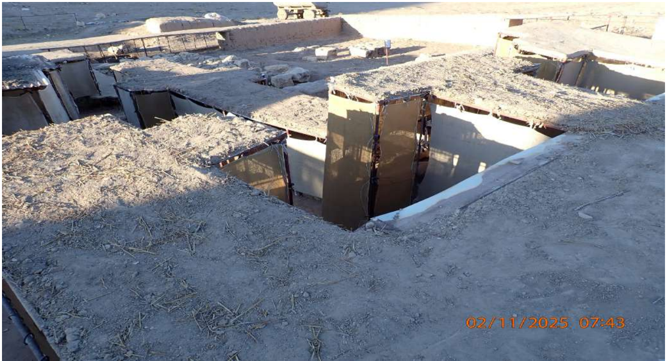
Figure 25: Preparation of service wing surfaces
